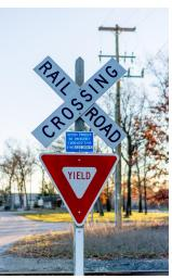
A passive railroad crossing does not have electronic warning devices, such as bells, gates or flashing lights. It will have a crossbuck, and a yield or stop sign.
